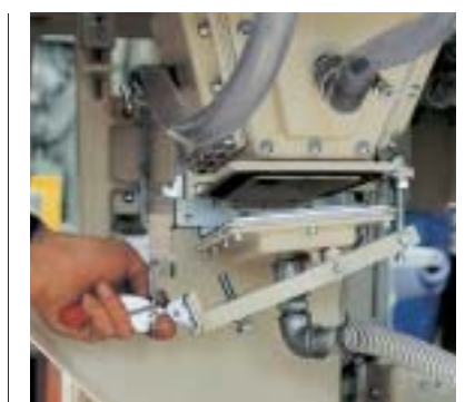
Maintenance door on the filling hopper
